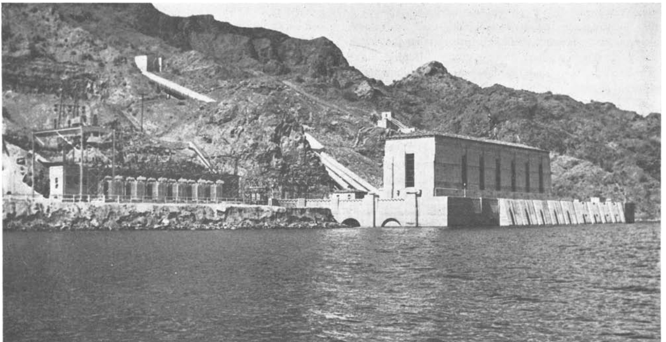
Lake Havasu reservoir is a stock pile of water for the Southern California area market. The building in the picture is the intake pumping station which starts the water on its way over the longest man-made aqueduct system in the world.
