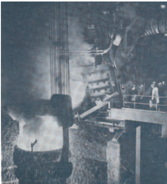
A modern high-powered 22 ft shell diameter Heroult furnace of 150 ton capacity. (Courtesy of the Lukken Steel Co.)
