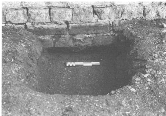
FIGURE 10. How not to construct a foundation for a two-storied building: two courses of brickwork straight onto clay. This is the northern wall of the southwestern gatehouse of the stables complex. Scale in 1 cm and 5 cm divisions. (Photograph by Graham Connah, 1997.)
