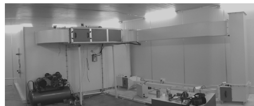
Fig. 1. Test system. (a) Experimental flowchart. 1, Window; 2, small chamber; 3, humidifier; 4, finned tube heater; 5, finned tube exchanger; 6, air-conditioning processing section; 7, wind pipe; 8 and 14, fan; 9 and 13, test chamber; 10 and 12, test section; 11, working section; 15, sampling pore. (b) Experimental system picture.
