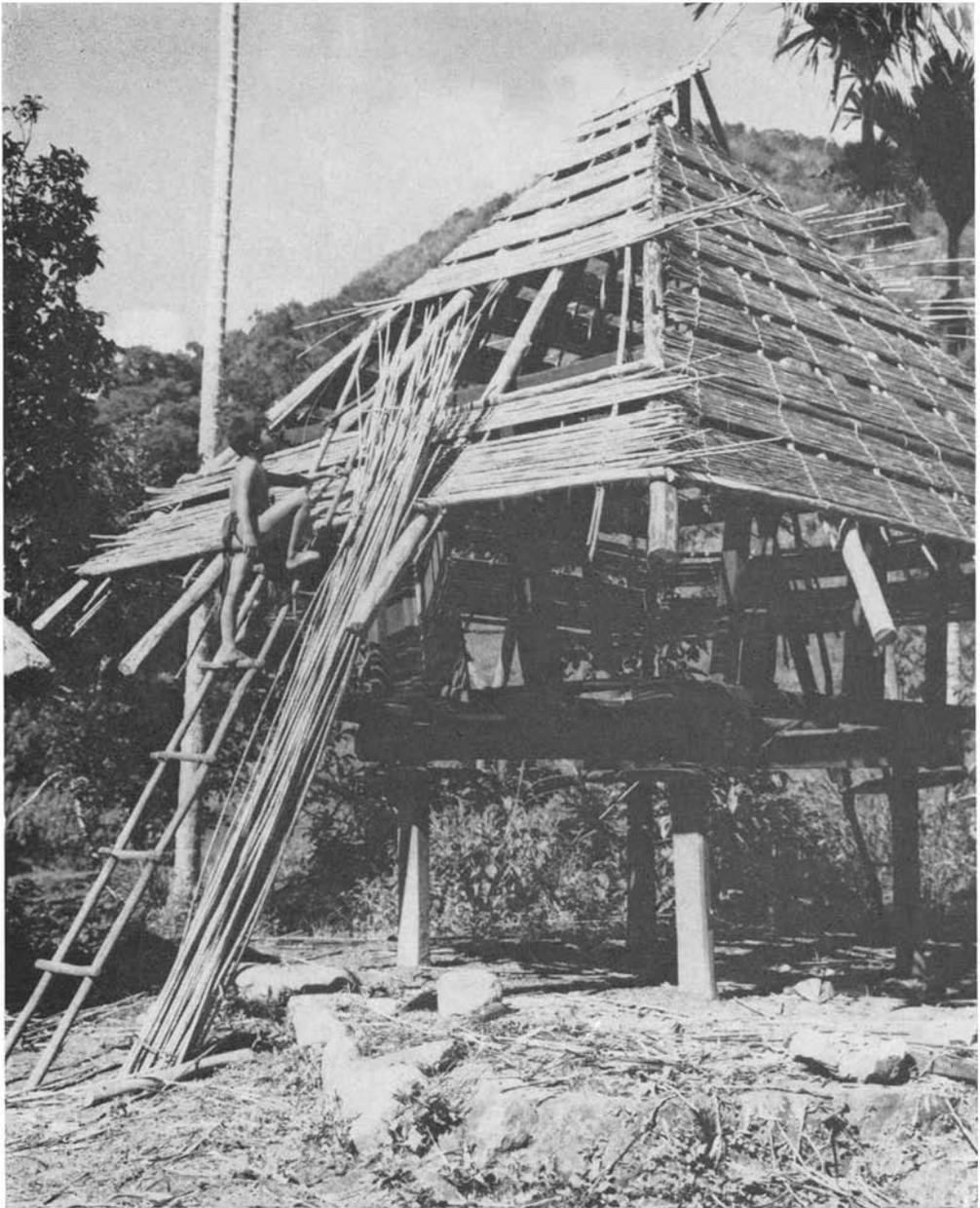
Fig. 3. Roof frame construction showing the use of *Miscanthus* cane grass (*bilâu*, [32; 42]) stems; Bayninan, 1962.
