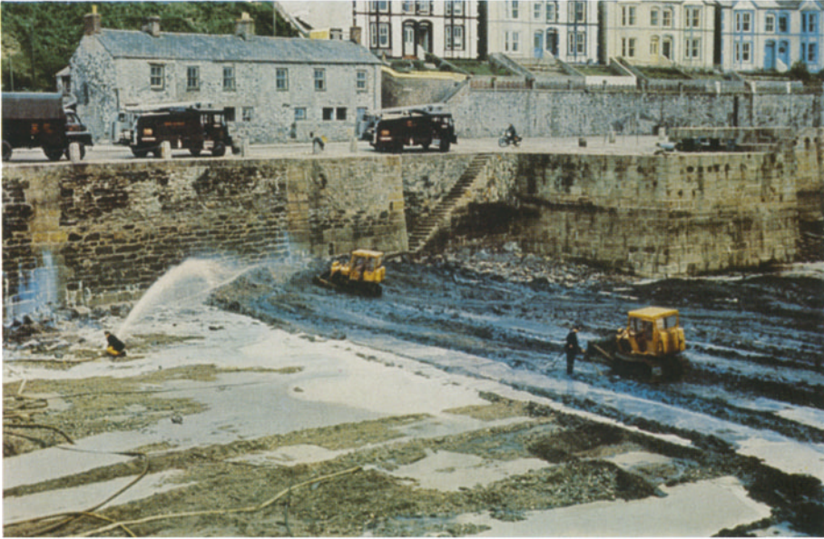
Fig. 8: Oil cleansing operations in Porthleven Harbour, 28th April, 1967. Bulldozing the harbour floor and detergent spraying the heavily polluted harbour wall. (Photo: P. E. GIBBS)
