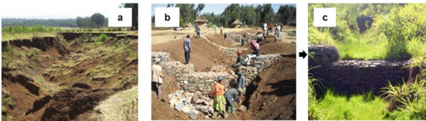
Fig. 9.13 Example of Ethiopia's common SWC measures; gully plugs constructed across gullies. a Gullies, b before (2012) and c after (2013) the interference. Source Haregeweyn et al. (2015)
