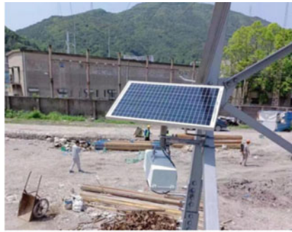
(b) Equipment installation
