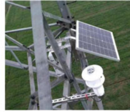
(b) Equipment installation
