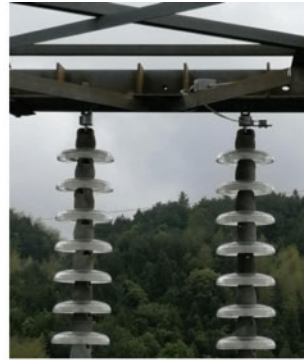
(b) Equipment installation
