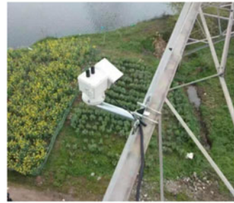
(b) Equipment installation
