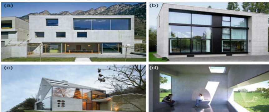
Fig. 2 a LWC: Schweiz 2003 (Gartmann house), with density 1,100 \text{ kg/m}^3 , strength 12.9 MPa, and thermal conductivity 0.32 \text{ W/m K} [50], b Infra LWC: Berlin 2007 (Schlaich house) with density 760 \text{ kg/m}^3 , strength 7.4 MPa, and thermal conductivity 0.18 \text{ W/m K} [51], c LWC: Stuttgart 2012 (house H36) with density 1,000 \text{ kg/m}^3 , strength 10.9 MPa, and thermal conductivity 0.23 \text{ W/m K} [50], d Infra LWC: TU Eindhoven 2015 (Pavilion) with density 780 \text{ kg/m}^3 , strength 10 MPa, and thermal conductivity 0.13 \text{ W/m K} [50]
