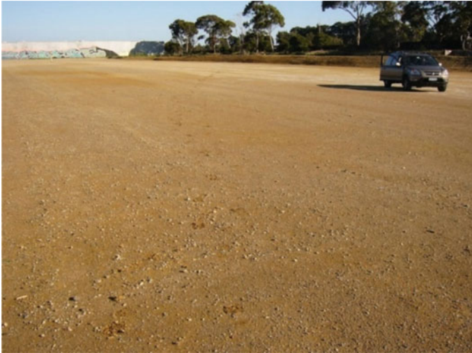
Fig. 8 Using enzyme as an additive for soil stabilization of a construction site consisting of 65,000 m 2
