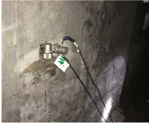
Fig. 9 Vertical acceleration sensor on tunnel side wall installed on site
