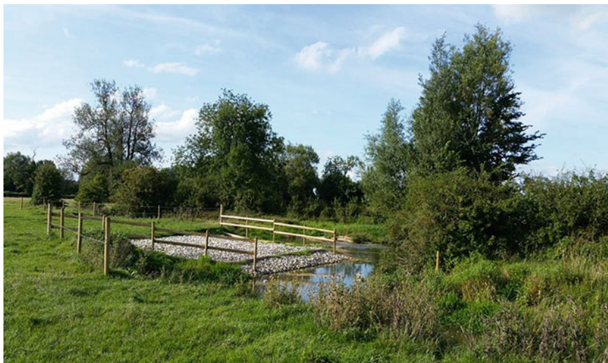
Fig. 9.4 Soil erosion mitigation measure (drinking bay) for cattle when accessing the river (photo: Jenny Phelps)
