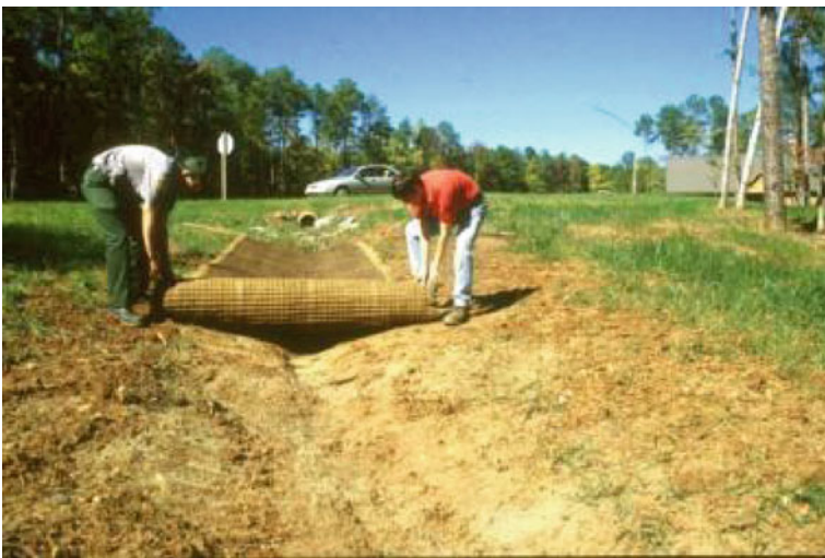
Turf Reinforcement Mats are an alternative to rock-line swales.
