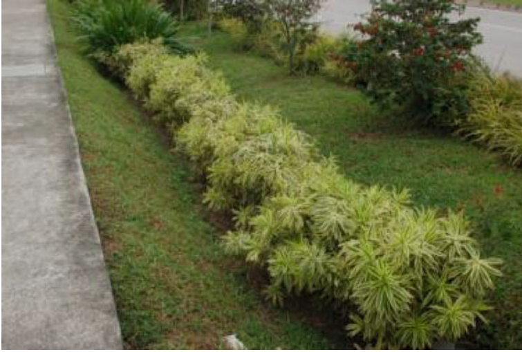
Example of a bioretention cells located along a streetscape
