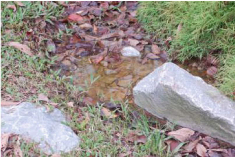
Water collected in a swale can become a mosquito habitat.
