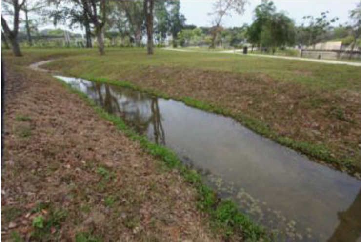
Maintenance of swales with collected water should focus on mosquito prevention.
