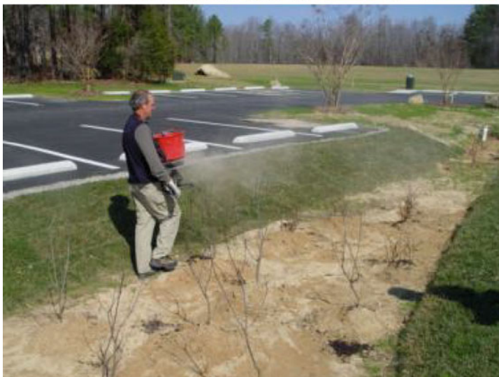
Various bioretention maintenance activities include: annual to semi-annual pruning (top), and an initial fertilization to ensure plant survival (bottom).
