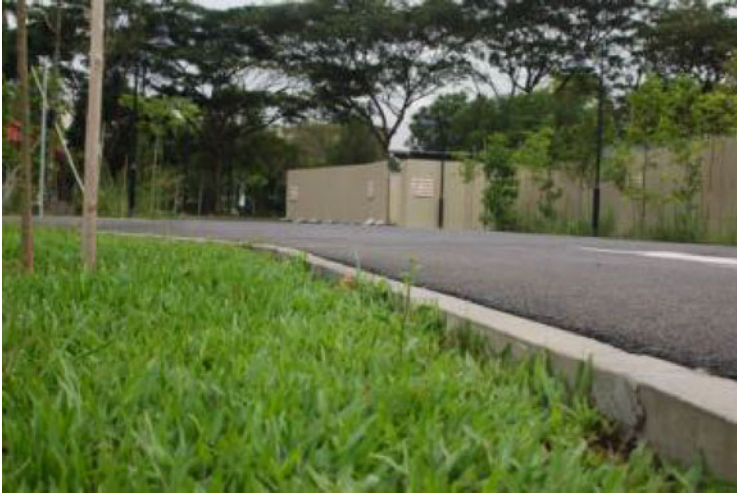
A 70-mm difference in elevation between pavement edge and turf grass reduces the risk of rill erosion.
