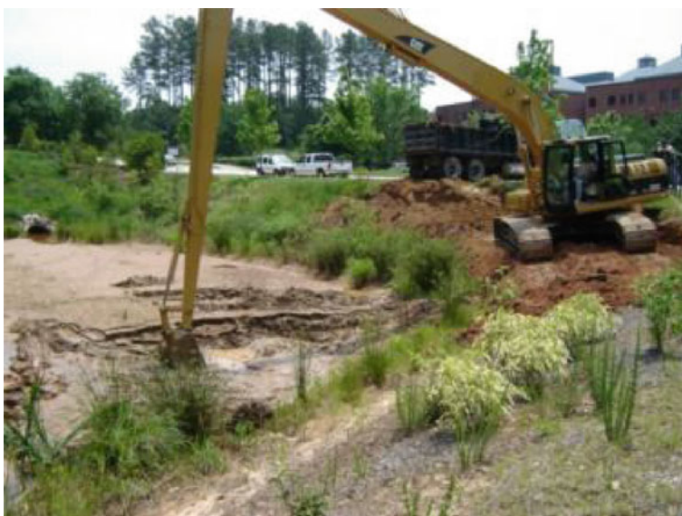
Cleanout is less frequent in stable catchments.
