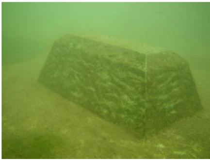
Photo 7. Attached algae on EAC panel
