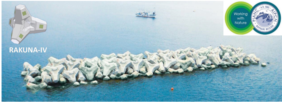
Photo 1. EAC Demonstration experiment in the construction of the 6 th breakwater at the port of Wajima (PIANC Working with Nature Certificate of Recognition)
