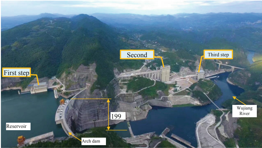
Fig. 9. Goupitan three-step ship lift in China
