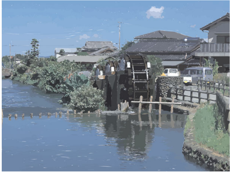
Fig. 3.8 Waterways and turbines (Fukuoka Prefecture)
