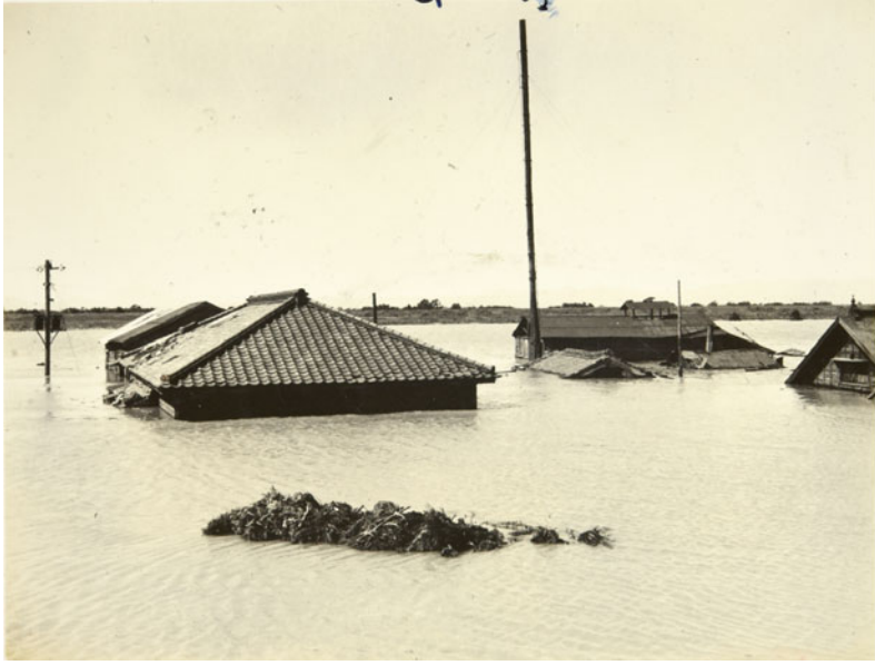
Fig. 4.28 Flood damage caused by the Kathleen Typhoon in September 1947. Arakawa River Basin, Suburb of Tokyo, A. Laflamme photograph collection, USAHEC. A. Laflamme was a photographer for the US Army Signal Corps
