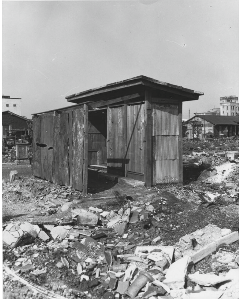
Fig. 4.17 A temporary toilet built in a burned-out area, November 3, 1945. Tokyo, Japan. US Strategic Bombing Survey (USSBS) photo. 243-GM-1G06. NARA
