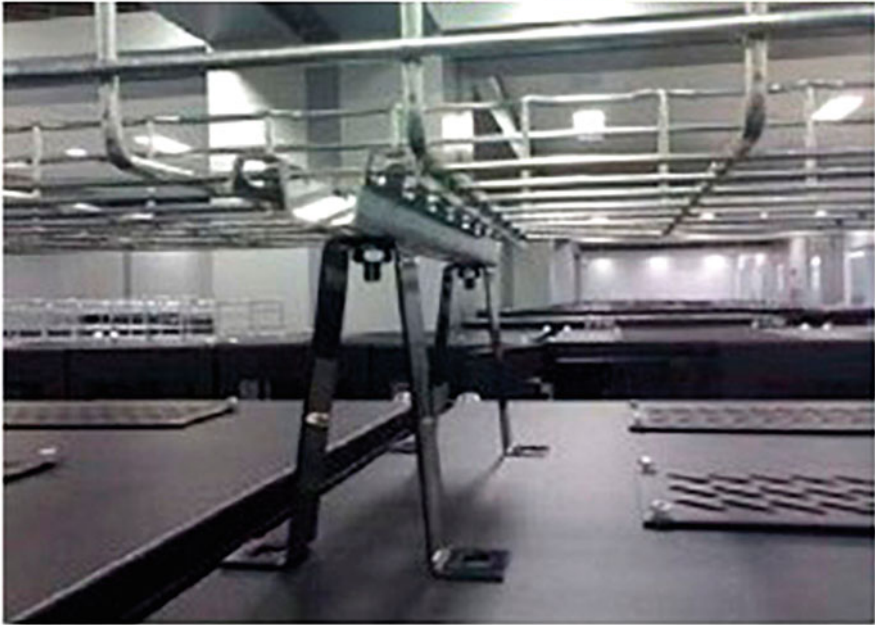
Fig. 2.64 Installation of supporting bridge for rack
