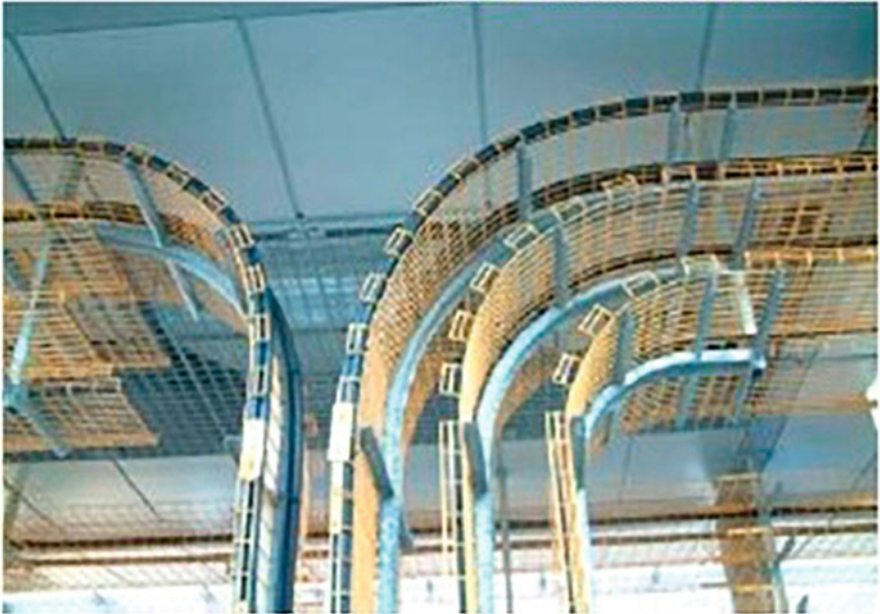
Fig. 2.63 Layered installation of bridges
