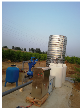
Fig. 4. The pressure spray equipment.
