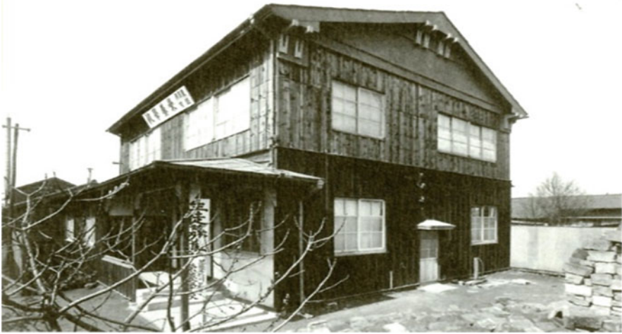
Photo 3.1 Saiki Nutrition School at the foundation (around 1924)
