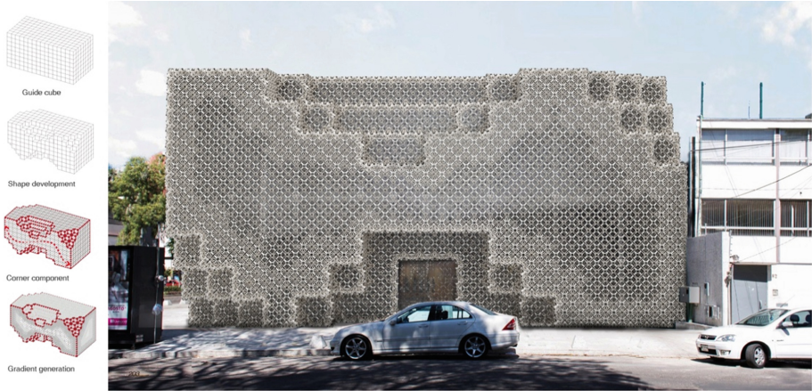
Fig. 24. Hybrid building structure generation
