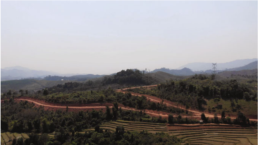
Fig. 1 Temporary access roads built for constructing remote segments and 109 tunnel portals of the China-Laos Railway. Consisting of both new construction and upgrades of existing tracks, these roads potentially increase connectivity among remote villages, but their maintenance beyond the opening date of the railway remains uncertain. Photo by Xiaoxuan Lu (March, 2019)
