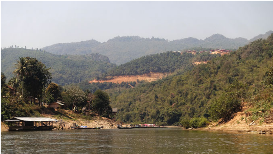
Fig. 7 Nam Tha River, a major tributary of the Mekong River, approximately two months before completion of a Chinese-funded hydropower dam 55 km downstream. This photograph shows: (1) an existing village (left) that will be inundated; (2) a newly constructed resettlement village (top-right) atop a ridge; and (3) a road (center) newly cut into the hillside, constructed above the soon-to-be reservoir draw-down zone. Photo by Jane Li Aijing (March, 2018)
