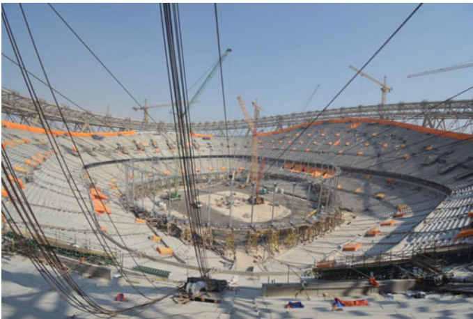
Fig. 7.2 The construction of the cable net roof
