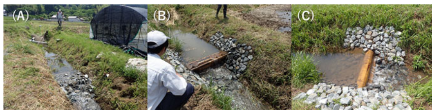
Fig. 12.5 Resulting structure of dams. Dams create permanent aquatic areas and step-pool structures in the channels. Dams were built using three types of materials. (a) Stonework. (b) Flashboard. (c) Log
