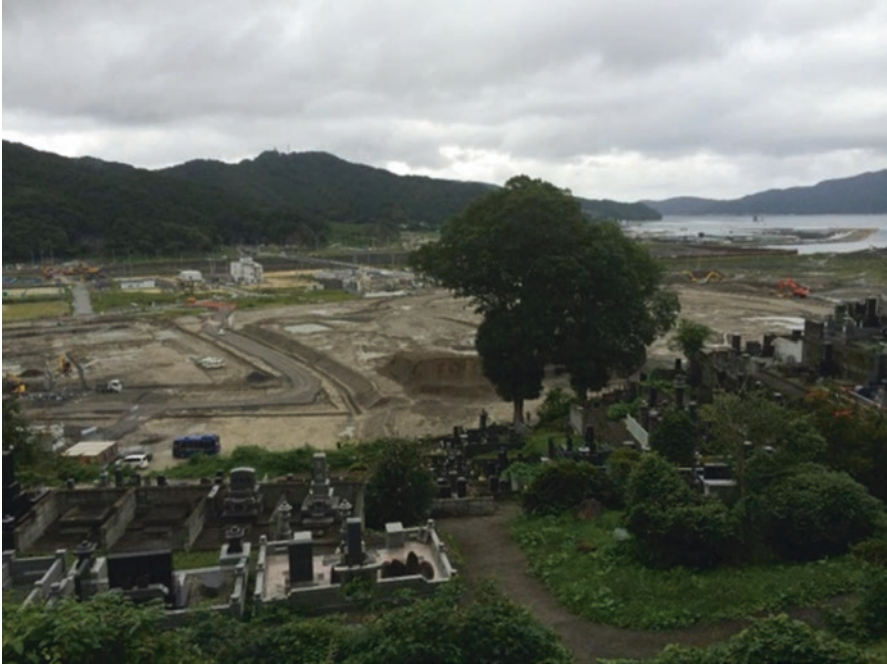
Fig. 7.2 The entire downtown area of Otsuchi is being elevated, as part of the strengthening of Layer 2 countermeasures
