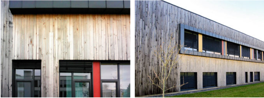
Fig. 5.2 Non-uniformly weathered building. Right image courtesy of Lone Ross Gobakken, NIBIO
