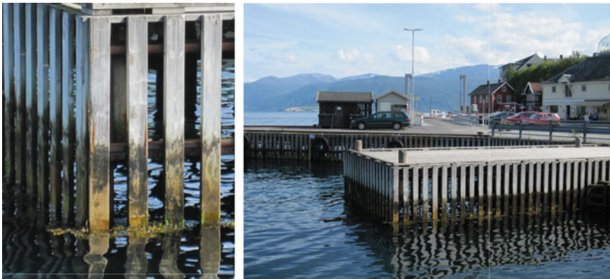
Fig. 5.9 Wooden pier exposed to fluctuations of the water level. Image courtesy of Lone Ross Gobakken, NIBIO
