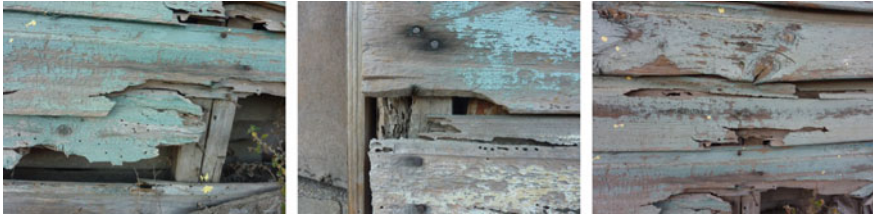
Fig. 5.10 Wooden façade degraded by insects. Images courtesy of Magdalena Kutnik, FCBA
