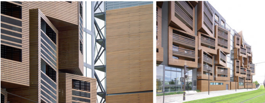
Fig. 2.15 Use of HPL in a building façade of Basket Apartments in Paris (OFIS Architects)
