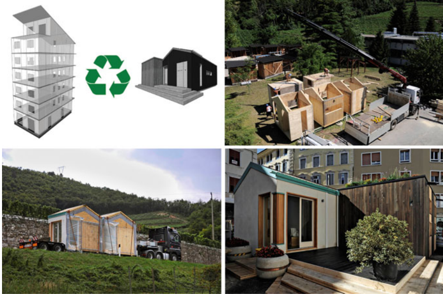
Fig. 2.24 Casa MAI as an example of a building constructed with reused cross-laminated panels. Image courtesy of Romano Magrone and Paolo Simeone—DUOPUU
