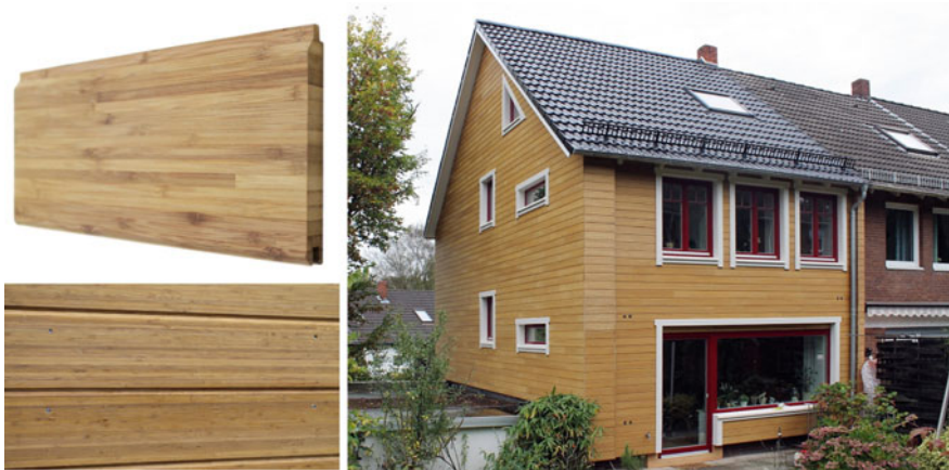
Fig. 2.12 Use of bamboo as a building façade material. Photograph courtesy of Kul-bamboo
