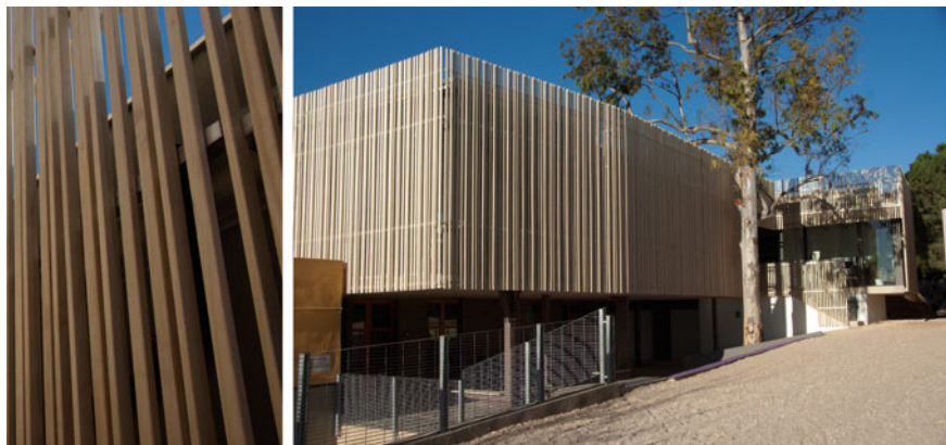
Fig. 2.8 Acetylated wood as a material for a building façade. Photograph courtesy of Accsys
