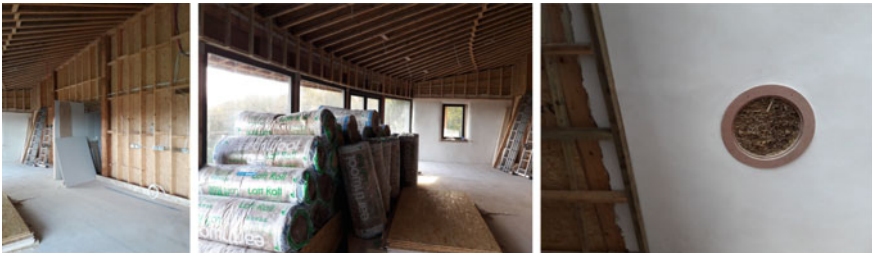
Fig. 2.6 Visitors' centre in Cuerden Valley Park Trust during the construction (November 2017)
