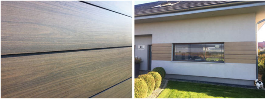
Fig. 2.14 Use of HPL as a building façade. Photograph courtesy of Ewa Osiewicz
