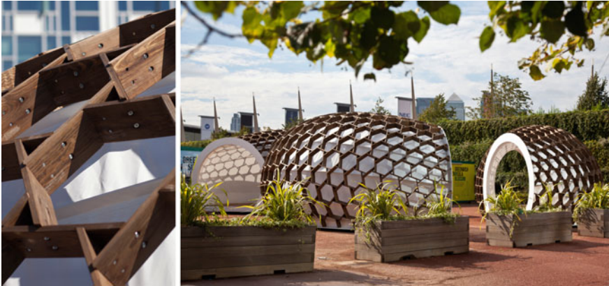
Fig. 2.9 Furfurylated wood as a material for a building façade. Photograph courtesy of Kebony
