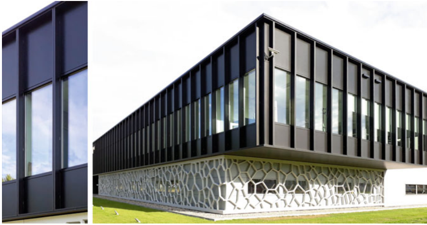
Fig. 2.11 Use of bio-based panels (Accoya® and MEDITE® TRICOYA® EXTREME) in the building façade
