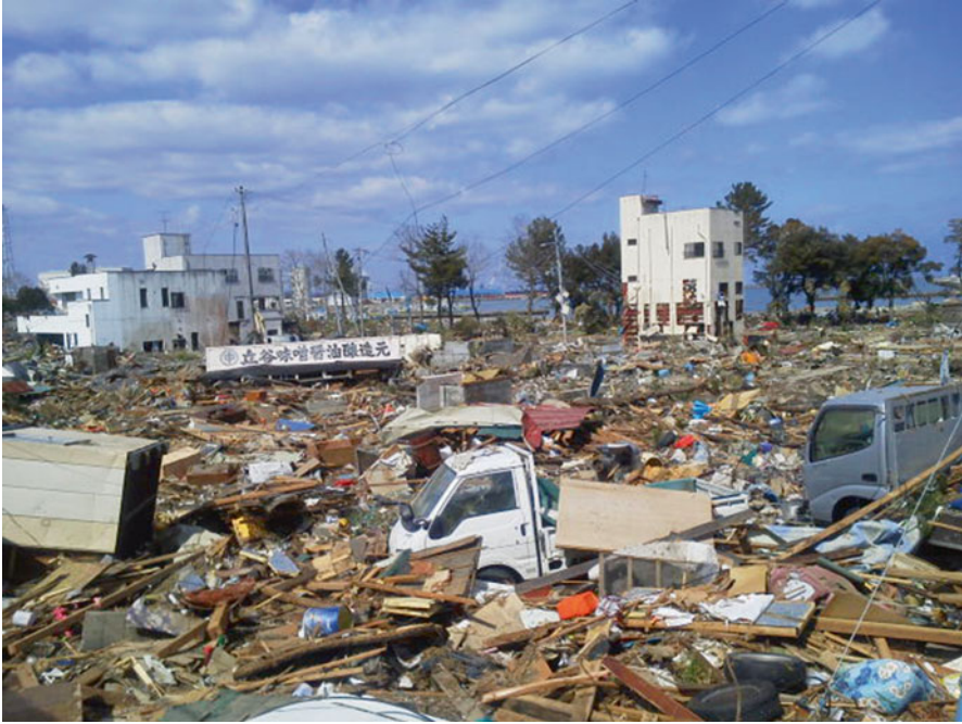
Fig. 1.1 The Haragama district, reduced to a mound of debris by the tsunami's onslaught
