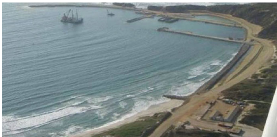
Fig. 13.11 Groins installed close to the Ehoala port
