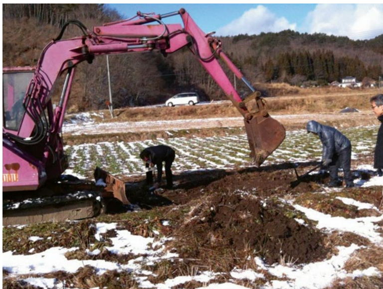
Fig. 13.5 Stripping the frozen soil using a backhoe by a local farmer on January 8th, 2012
