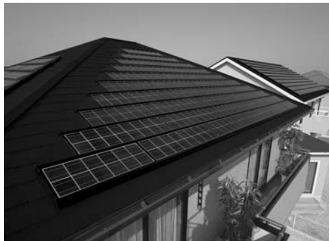
Fig. 6-3: Solar cells installed on a roof of a house (Courtesy of KYOCERA Solar Corporation)
