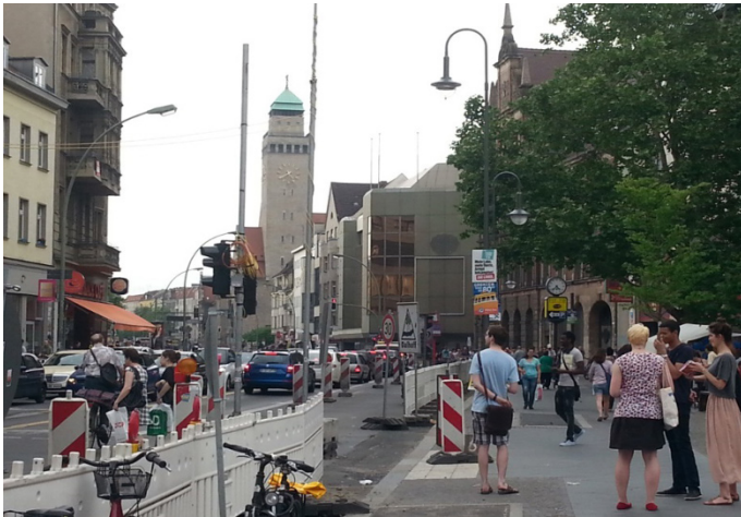
Fig. 10 Crowded sidewalk with construction site on Karl-Marx-Straße
