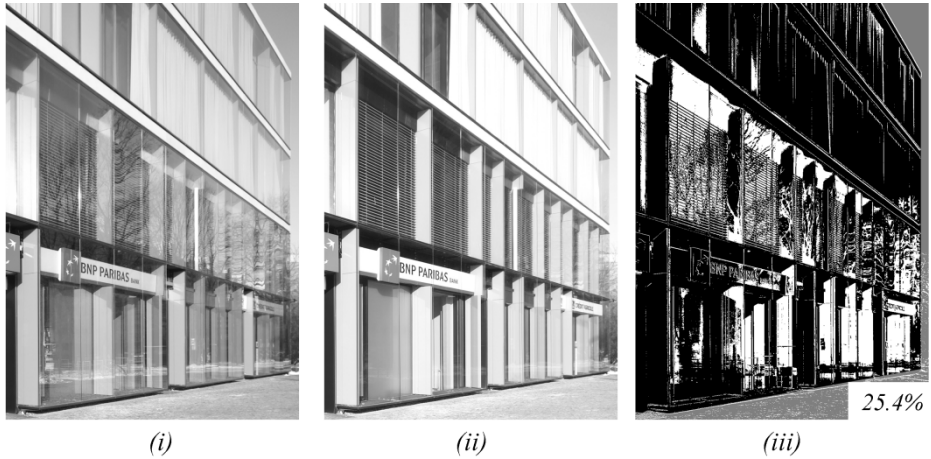
Fig. 3. Pictorial image analysis of series 2: (i) unmodified image, (ii) modified image with reflection filtered out, (iii) image thresholding and percentage calculation. Pictured building: the Thespian Housing and Office Building (by Mackow Pracownia Projektowa, 2012)
