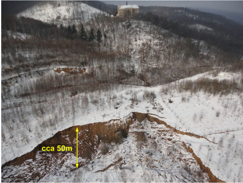
Fig. 7. Landslides at the pillar protecting the castle [11]
