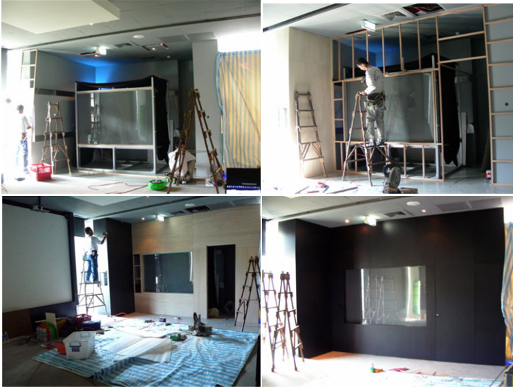
Fig. 2. Interior design construction of 100-inch multi-touch display
