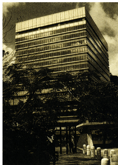
212 The offices of Springer-Verlag Hong Kong are located on the seventh floor of the Mirror Tower on Kowloon Peninsula.
