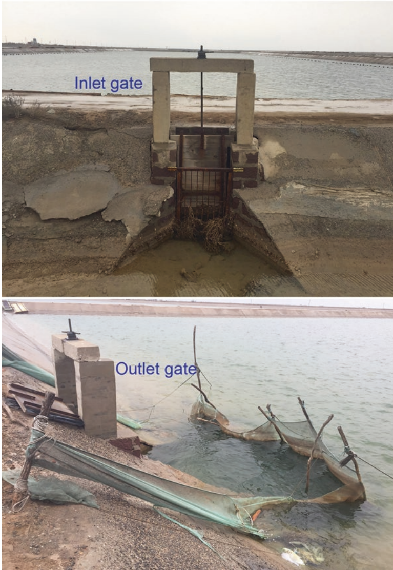
Fig. 4.4 Inlet gate with channel higher than water level; and outlet gate with channel lower than water level. (From Mao)
