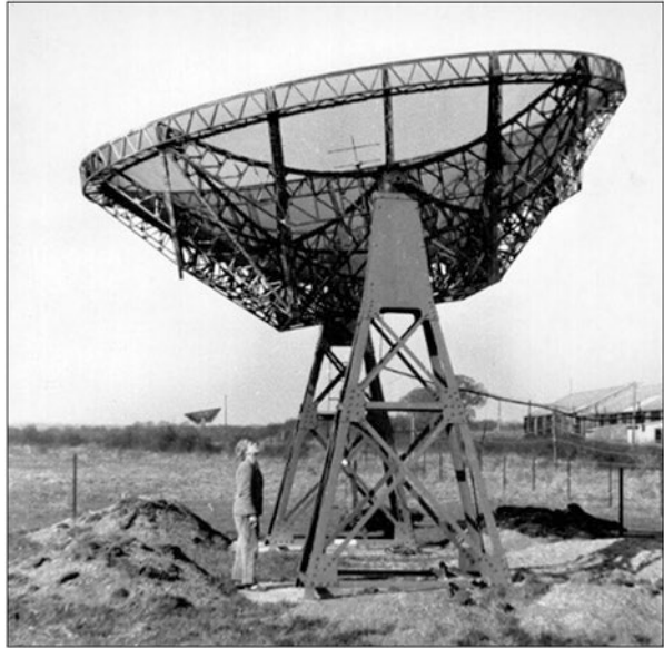
Fig. 2.10 Graham Smith with one of the 7.5 m diameter Würzburg dishes used in the interferometer at Cambridge for accurate measurements of radio source positions (courtesy: Robertson collection)
