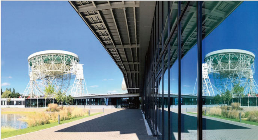
Fig. 5.31 The SKA Organisation is housed in a new building at Jodrell Bank. The organisation planning the world's largest radio telescope is next door to the very first giant radio telescope, completed in 1957. In 1987 the 250 ft dish was renamed the Lovell Telescope in honour of Sir Bernard. In February 2021, the SKA Organisation was superseded by the SKA Observatory, with Philip Diamond as the inaugural Director-General. The SKA Observatory is the intergovernmental organisation that will build and operate the SKA telescopes (courtesy: SKA Observatory)
