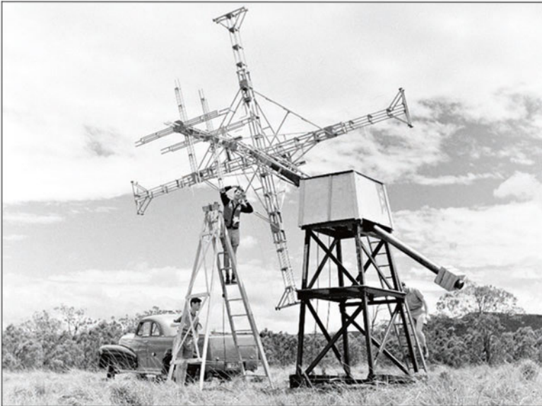
Fig. 2.47 (above) The Dapto field station showing the three rhombic antennas and the main receiver building. (below) The rhombic antennas were mainly made of wood. Their crossed rhombic configuration allowed polarisation measurements to be made of the solar bursts (courtesy: CRAIA)
