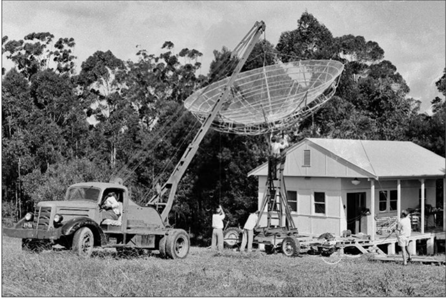
Fig. 2.68 Installation of the 6.4 m parabolic antenna and adjacent receiver hut at the Murraybank field station. This site in West Pennant Hills was located on an orchard belonging to John Murray's father, and so the name Murraybank (courtesy: CRAIA)
