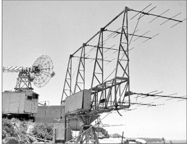
Fig. 2.20 The 8-Yagi antenna was built at the end of 1951 and installed on an old wartime mount a little to the south of the blockhouse and close to the cliff edge (courtesy: CRAIA)
