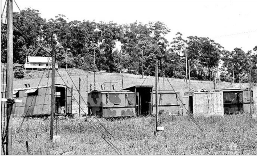
Fig. 2.29 The Hornsby Valley field station showing the antennas, transmission lines and instrument huts used by Kerr, Shain and Higgins in the 1948 Moon-bounce experiment. Radar signals at 17.84 and 21.54 MHz were transmitted from Shepparton (Victoria), bounced off the Moon, and received at Hornsby Valley (courtesy: CRAIA)
