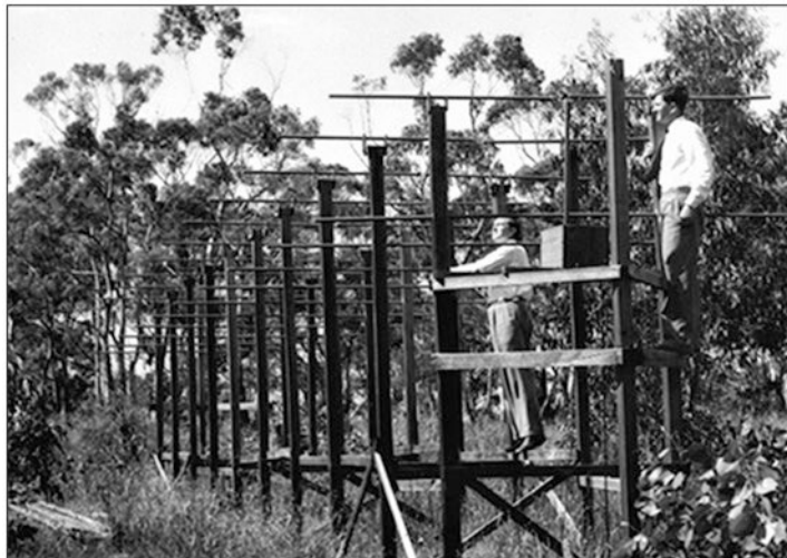
Fig. 1.41 The mechanically phase-switched 100 MHz interferometer built around 1952 at Mount Nelson, Hobart, by Gordon Newstead (shown at right) from the Department of Electrical Engineering at the University of Tasmania (courtesy: Martin George)
