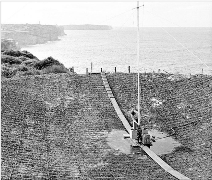
Fig. 2.22 The original 22 m 'hole-in-ground antenna', one of the largest radio telescopes in the world, was built by the Dover Heights staff as a lunchtime project in 1951. The catwalk provided access to the centre of the dish, the aerial mast and dipole, and the instrument box at the base of the mast that contained part of the 160 MHz receiver (courtesy: CRAIA)
