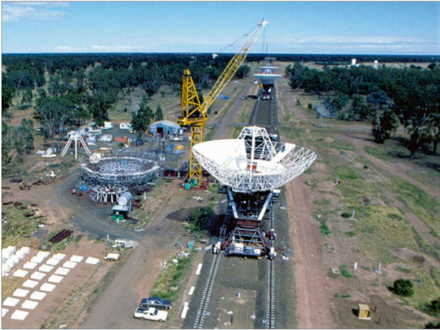
Fig. 5.14 The Australia Telescope Compact Array (ATCA) under construction at Culgoora in 1987. The extraordinary surface accuracy of each 22 m dish enables the array to operate at wavelengths as short as 3 mm (courtesy: CRAIA)
