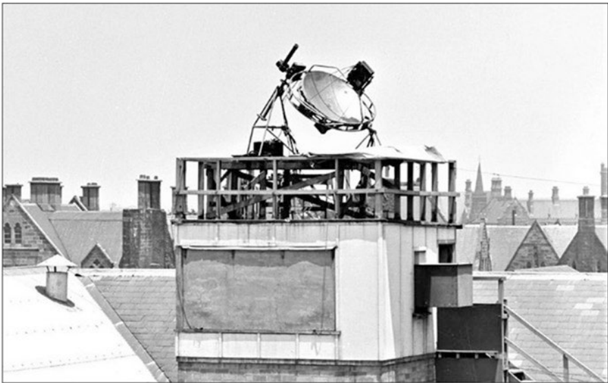
Fig. 2.9 The 'Eagle's Nest' was a small flat-roofed room at the very top of the Radiophysics Lab that was used for research and to test new equipment. Piddington and Minnett used the 1.1 m antenna to observe the Sun and Moon in 1948 (courtesy: CRAIA)
