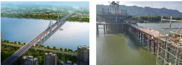
Fig. 2. Overview of the main span of Chaibu Bridge
