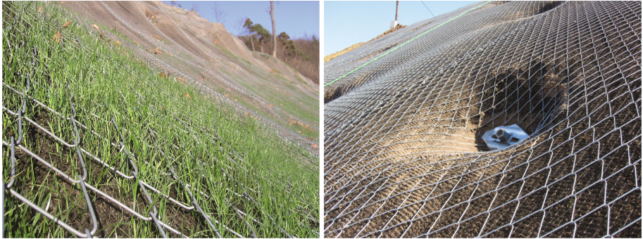
Fig. 1. TECCO® mesh and system spike plates
