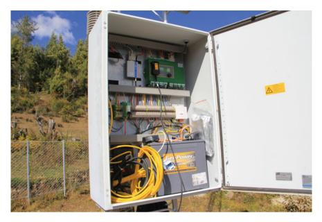
Fig. 2.3 Rara Nepal. OTT data logger and data transmission modem in IP65 enclosure
