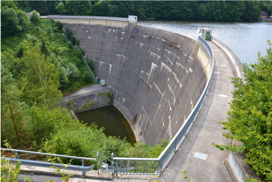
Fig. 3.13 A hydropower storage dam collects water continuously but produces hydropower only at times where there is specific demand, e.g. when wind and solar energy are insufficient. In contrast to a pumped-storage hydroelectric power station there are no pumps installed to pump up water in times of overcapacities and low demand [57]
