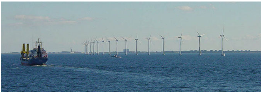
Fig. 3.5 Offshore wind farms, here in the vicinity of Copenhagen, have a large future potential due to the strong and less volatile winds and the almost unlimited space for wind farms [19]
