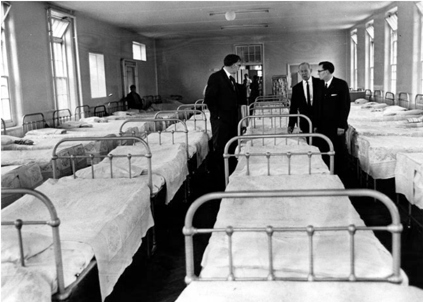
Fig. 7.1 Officials inspect a men's ward at Ely Hospital, 1969.
