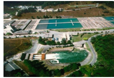
Fig. 2. The water treatment plant used for modelling and simulation
