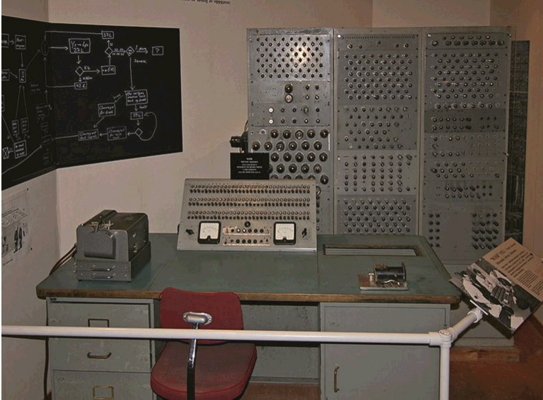
Fig. 6. NUSSE Norway's first computer derived from Booth's design 1954
