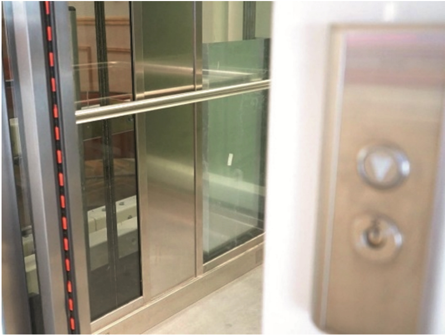
Fig. 3. Elevator at CDG airport in Paris. Elevator issues green LED light inside of the door while opening and red light while closing. Sensors are present so that passenger is not hurt if coincidentally present in the area of door closing.
