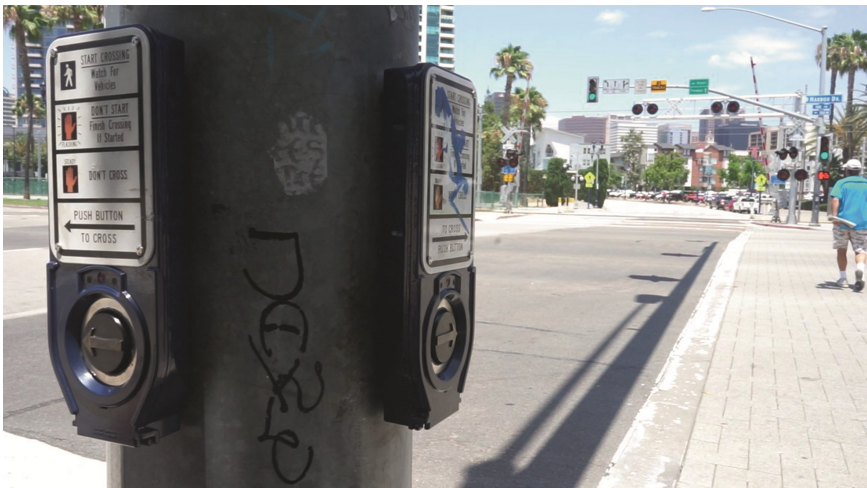
Fig. 4. A crosswalk in San Diego, CA. Implicit information on the time remaining for crossing the street by pedestrian is issued and visible for both, the pedestrian and driver of a car. Audible information is employed and counting the time remaining, which is especially beneficial for blind citizens. Feedback after pressing the request button is provided by audibly and visually.
