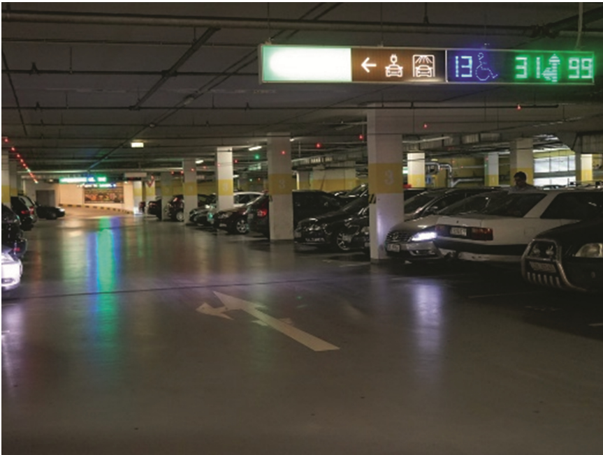
Fig. 2. Garages of the mall at Chodov subway station in Prague. Sensor above every carport reports the number of overall free position in the garage and its approximate position.
