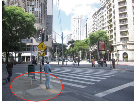
Fig. 4. Low floor and tactile floor indicator Low floor and tactile floor indicator can be very useful for people with reduced mobility/wheelchair users and visually impaired people. Yet, as shown in Fig. 4, sometimes they float on the sidewalk: no signs show how to reach them – especially to blind people.
