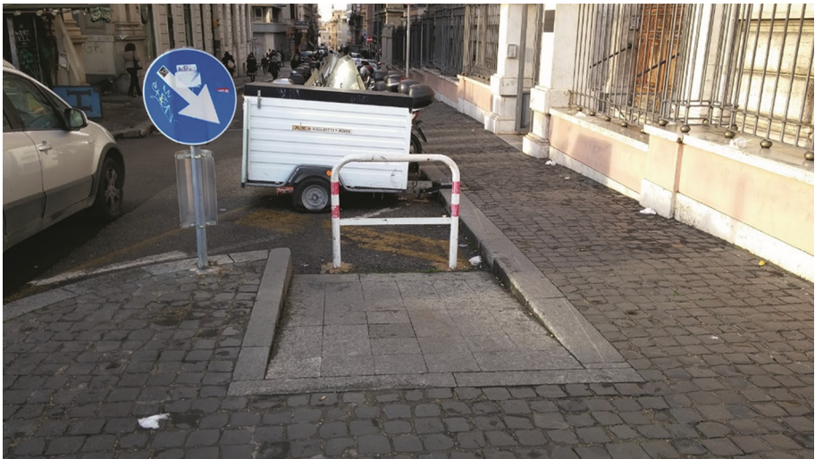
Fig. 4. One of the architectural barriers of the city of Rome
