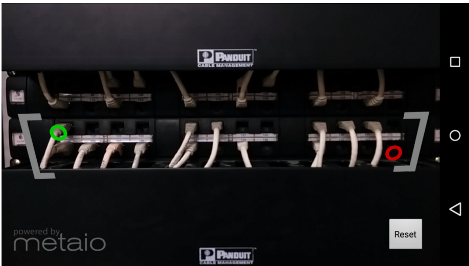
Fig. 3. A screenshot of the application used to support maintenance of network elements
