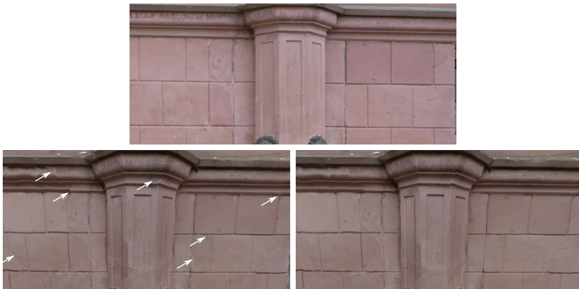
Fig. 12. Top row: One of the input images. Bottom row: Reconstructed City Wall color adjusted without support region and without Poisson editing, and the same reconstruction adjusted with support region and Poisson editing. (Best viewed on screen.)
